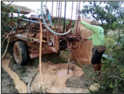
Figure 3 Water well being drilled for groundwater data ( https://li01.tci-thaijo.org/index.php/TSAEJ/article/view/251548class= )
